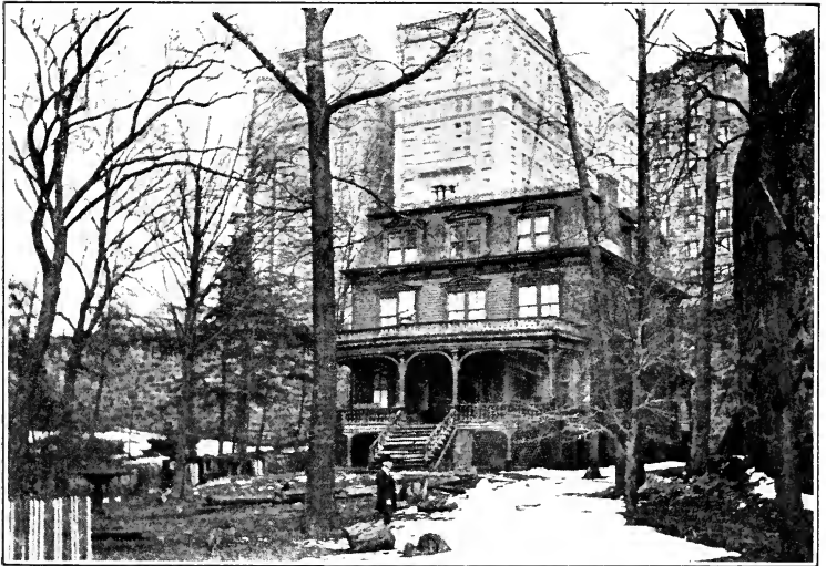
"MINNIE'S LAND" AS IT APPEARS TO-DAY FROM THE RIVER FRONT, POCKETED BY THE RETAINING WALL OF RIVERSIDE DRIVE.
